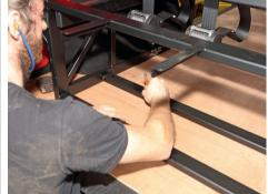
Once vou're happy the frame is in the right place, mark the fixing points on the floor using the pre-drilled holes in the bed frame. There are six in total
